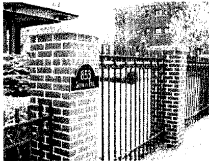
Square pillar with segmented cap.
