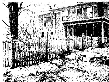
The step down of a fence to accommodate grade change.
