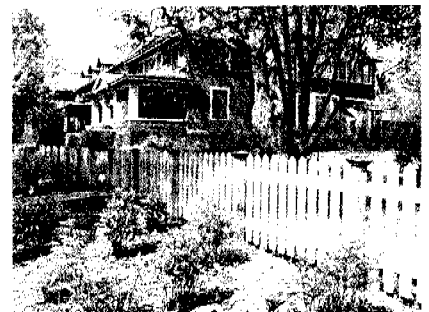
Posts should not be hidden by the pickets.
