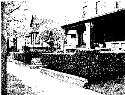
Low retaining wall.
