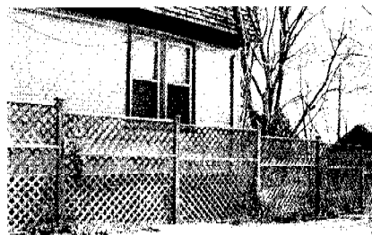
The step down of a fence to accommodate grade change.
